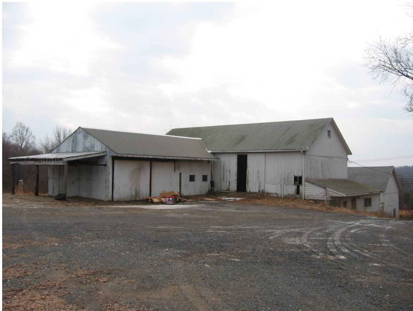
Figure 8 – The “upper” barn.
