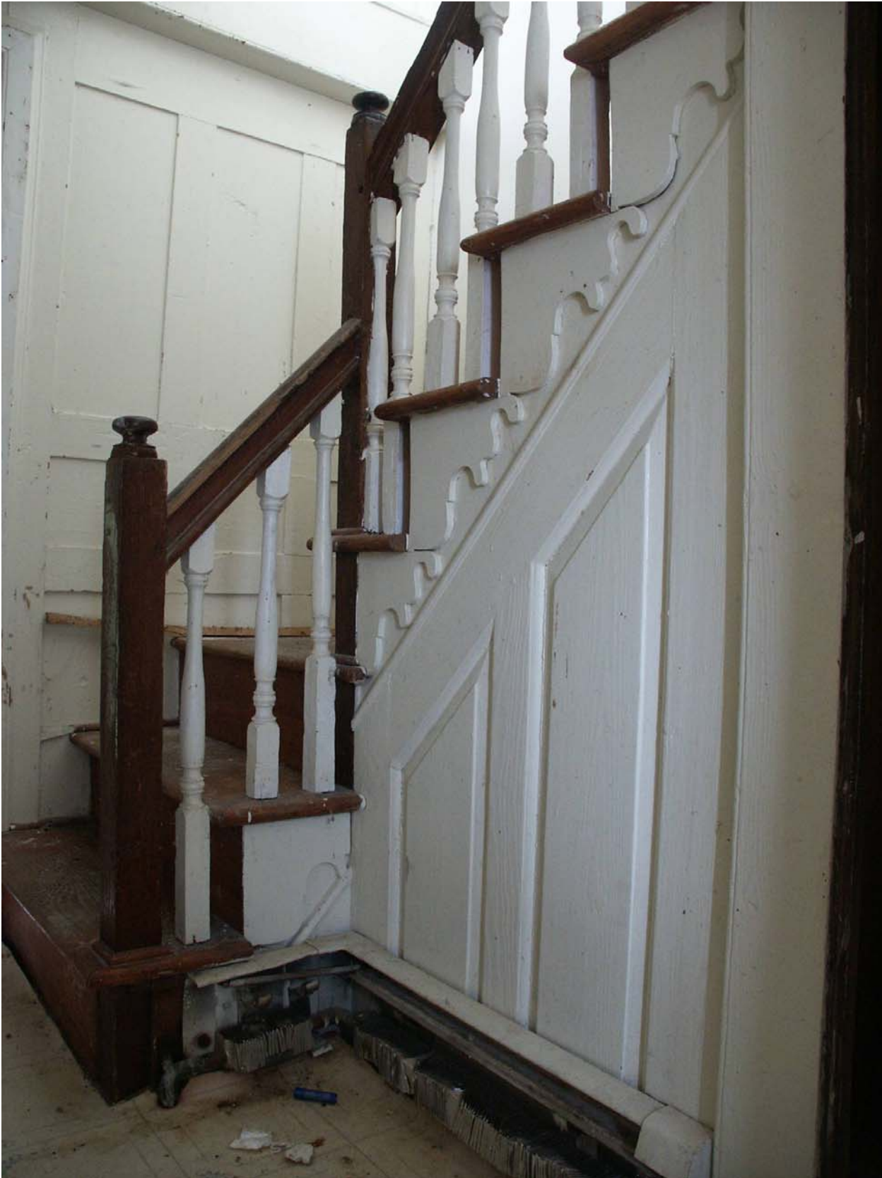
Figure 4 – The front stairs from the southwest.
