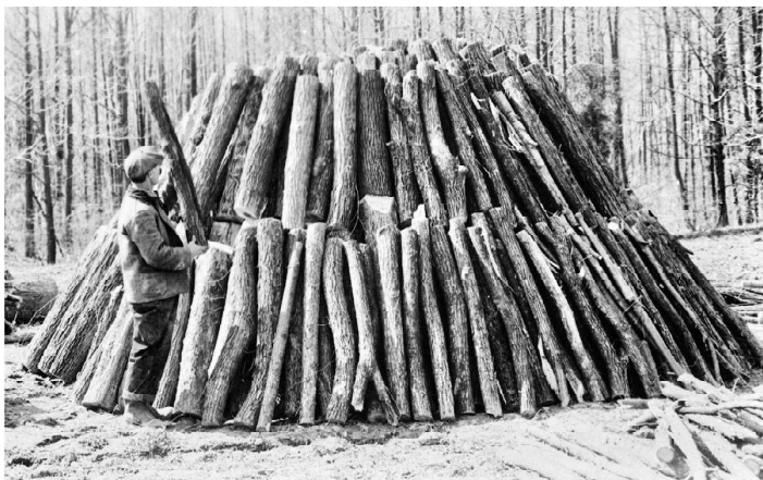
Image from Library of Congress, Historical American Buildings Survey, print borrowed from New Jersey Department on Conservation and Development, Charcoal Pit Prior to Burning, Lakehurst, NJ.
